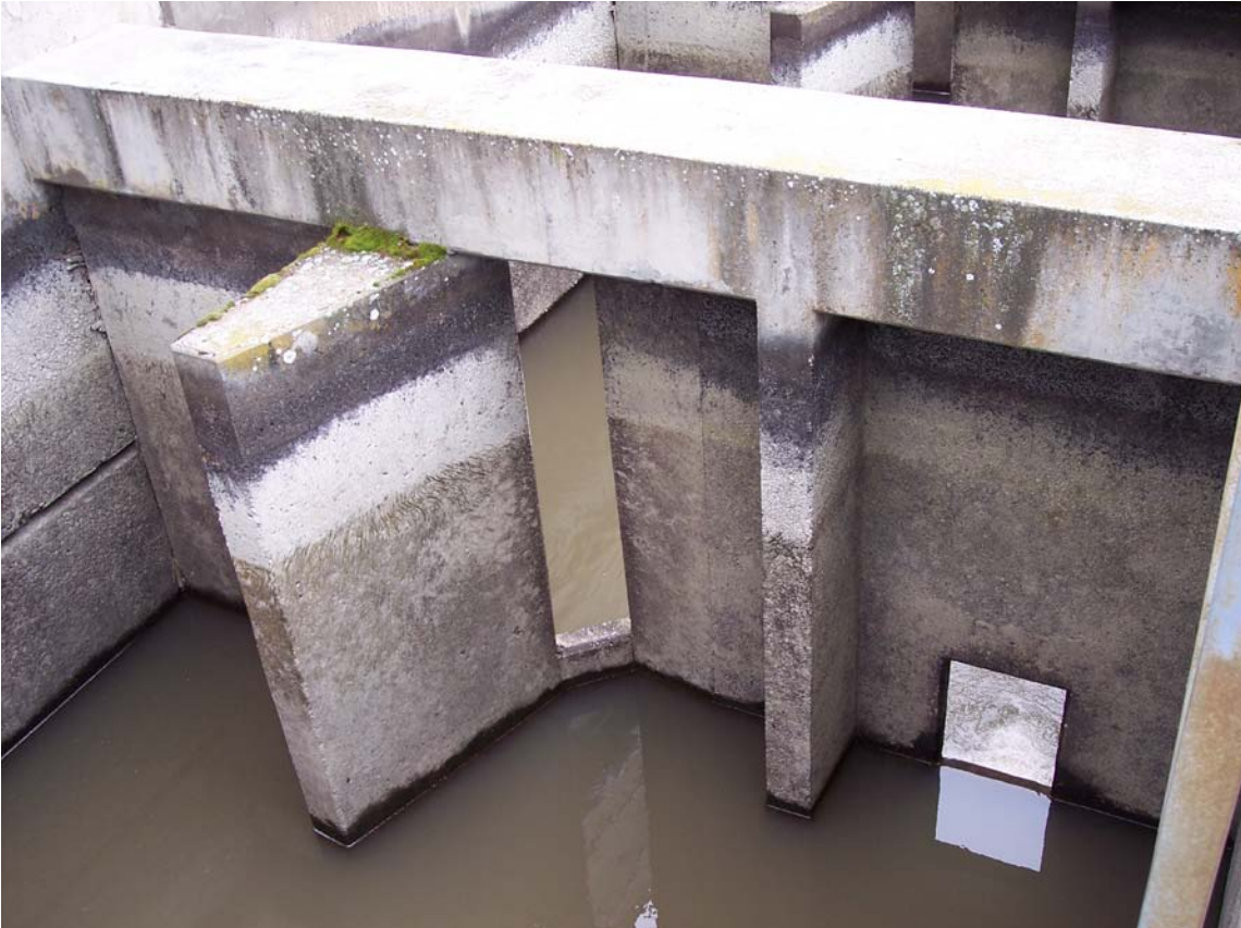
Figure 16 – North Shore Fish Ladder Control Section Typical Weir, Looking Downstream.
