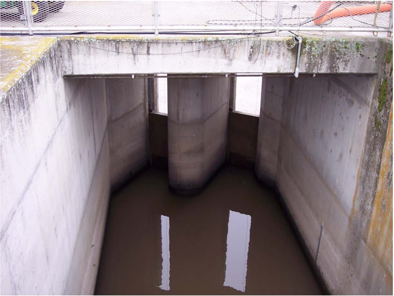
Figure 3 – North Shore Entrances NSE1 and NSE2 Looking Downstream.
