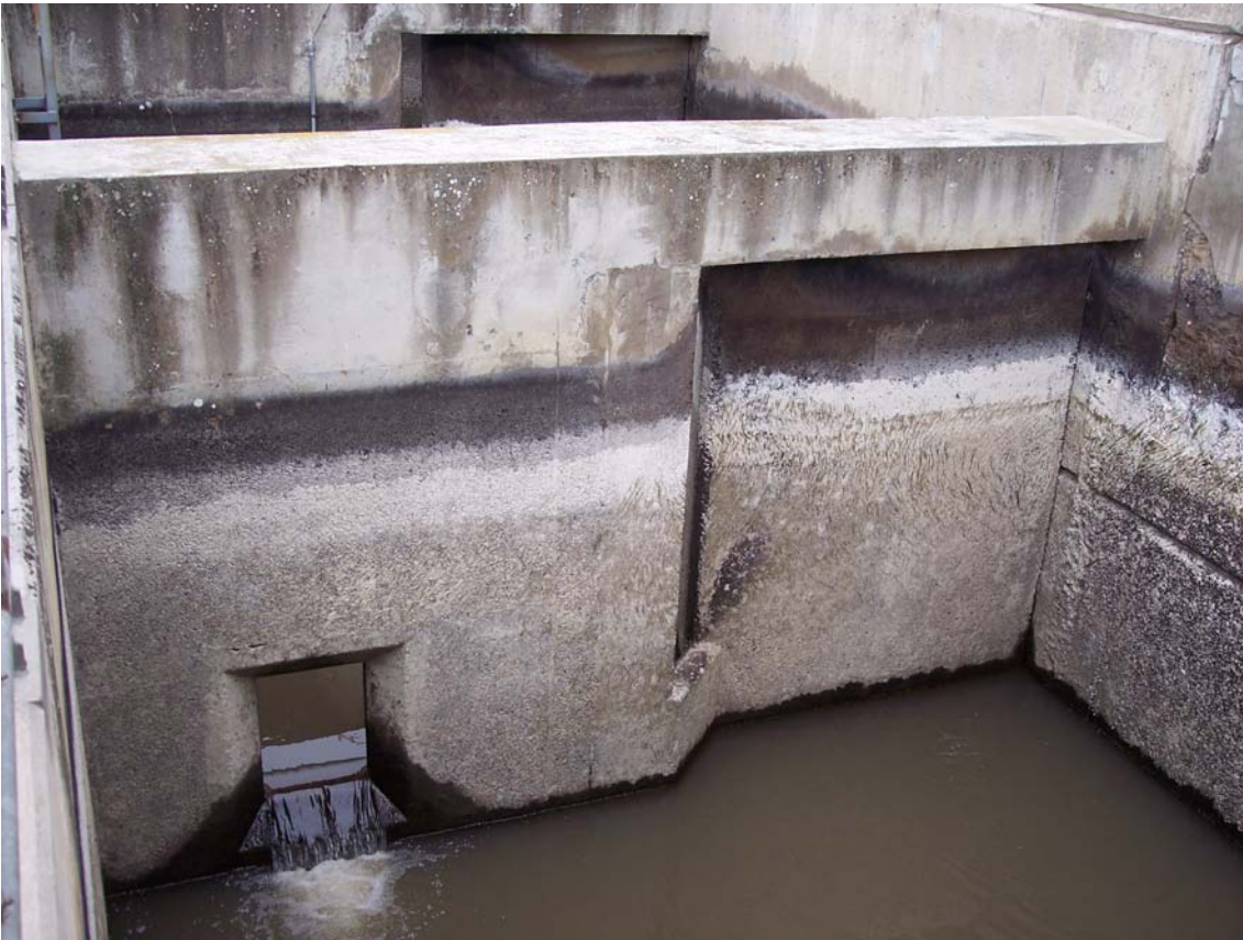
Figure 15 – North Shore Fish Ladder Control Section Typical Weir, Looking Upstream.
